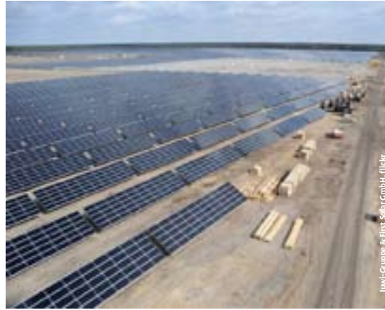
Solar energy park Lieberose
